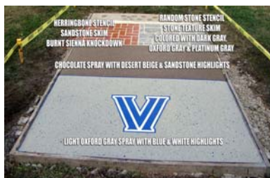
FIG. 8 DCO on outdoor field slab
