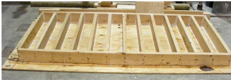
FIG. 1. Beam formwork
